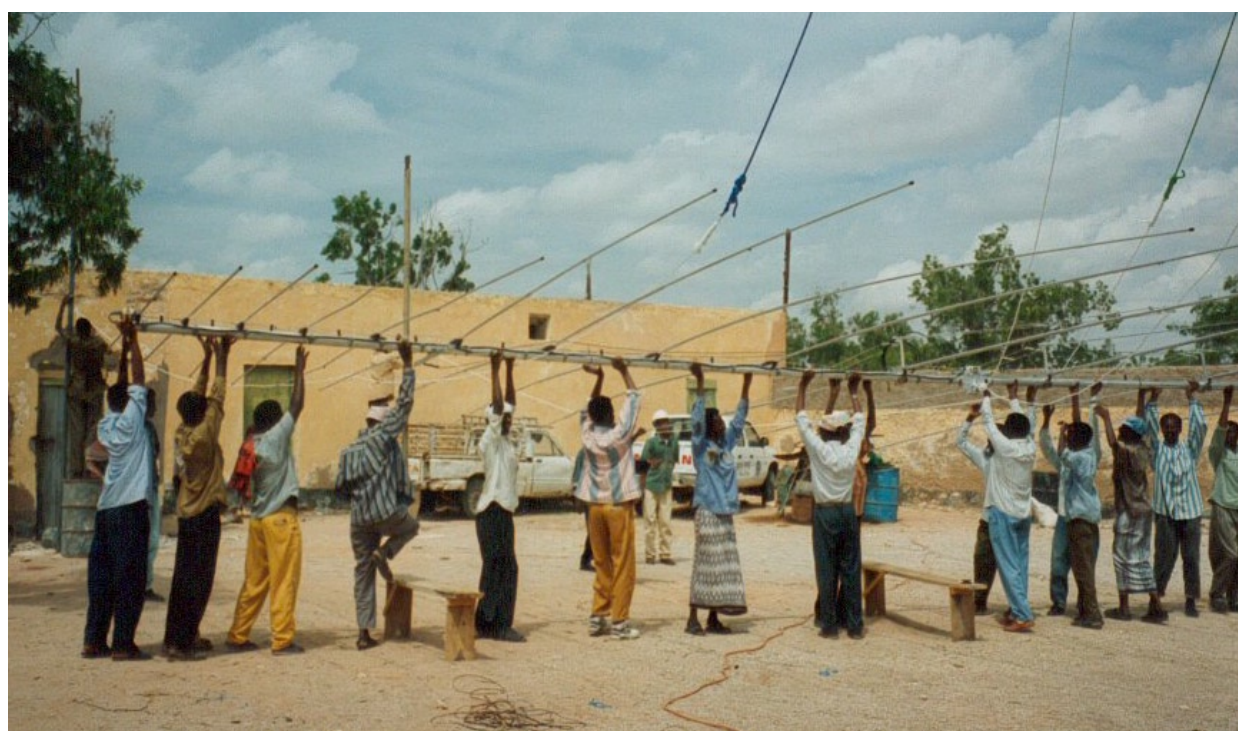
The antenna goes up!
